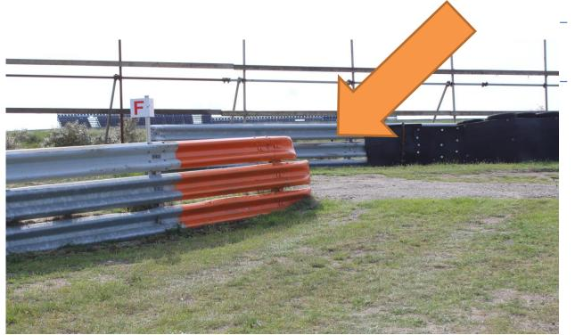
An orange armco means an opening in the guardrail.
